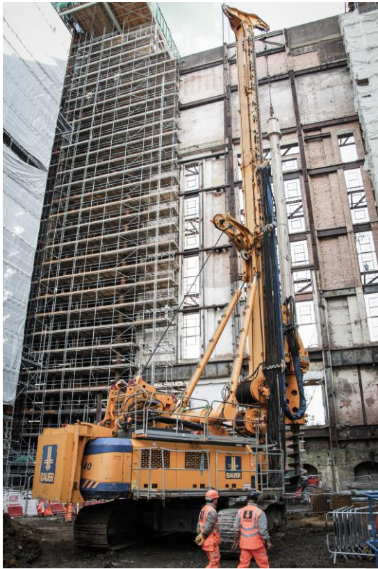
Bauer Technologies on site at Battersea
