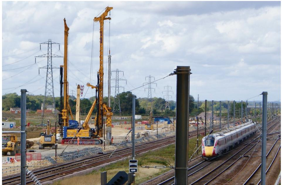
working rigs and cages were either taken in with line blocks or during night-time possessions. The Stamford UB allowed for small plant and pedestrian access to the worksite.
