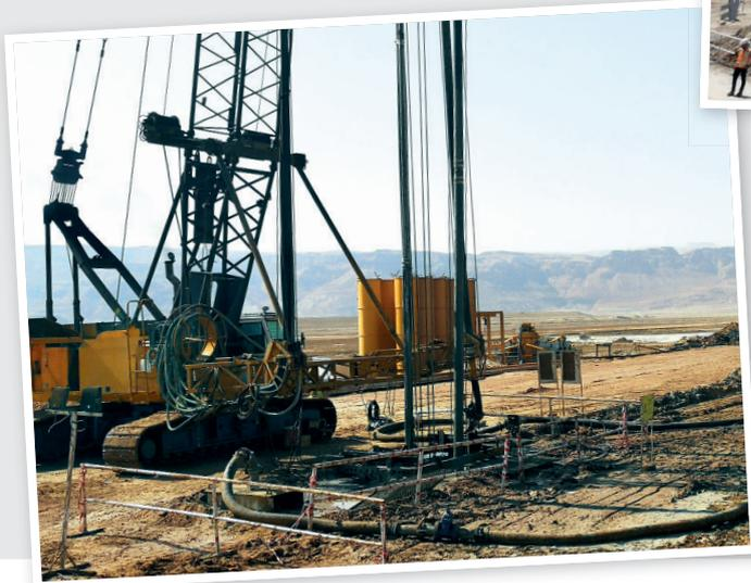
The cut-off wall, with a thickness of 600 mm, reaches between 18 m and 30 m into the ground.
