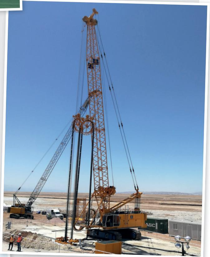
A total of 112,000 m<sup>2</sup> of cut-off wall with embedded sheet pile wall were constructed.
