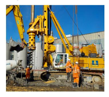
The work was undertaken with the chemical plant in operation, so the project team faced several challenges. Bauer had to install a number of rotary bored piles in close proximity to BASF's existing chemical storage tanks, carrying inherent risk, as well as influencing construction sequence.
