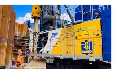
Specifically, Bauer was contracted to instal 4 no. x 54.5 m 1000 mm rotary bored piles, using 37 m of 1180 mm casing. These piles were crucial for supporting the abutment of the access road flyover bridge, over the depot access road, mitigating potential settlement issues due to back-filled mine workings in the area.
