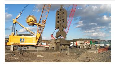
Bauer Technologies executed a circular shaped diaphragm wall and foundation barrettes for the facility in Newhaven for Hochtief UK.
