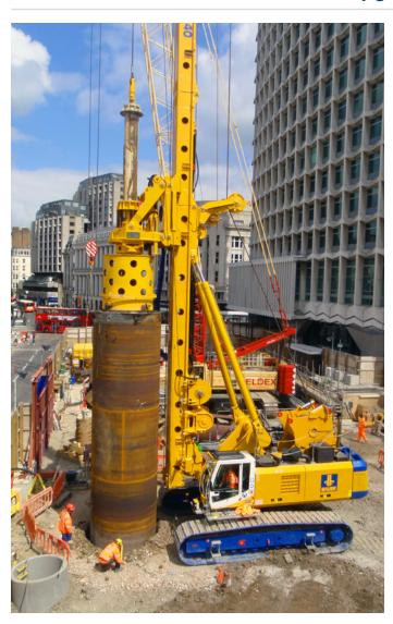
Bauer Technologies performed large diameter (2 m+) piling to below 65 m depth; diaphragm walling 1 m thick x 41 m deep; 11 no. plunged columns installed into large diameter 48.5 m deep piles; piles of diameter 2.4 m and various secant pile walls for main contractor Vinci / BAM Joint Venture, on behalf of the client, London Underground Limited.
