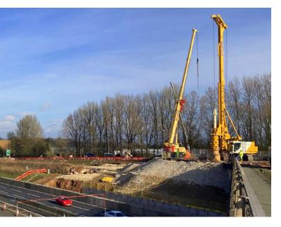
Bauer's scope of work was the installation of rotary bored piles for the A533 bridge replacement. All permanent piles in the new structure were 1180 mm dia., with drilled rock sockets into the underlying mudstone of varying lengths, to function as bearing piles for the new bridge structure.
