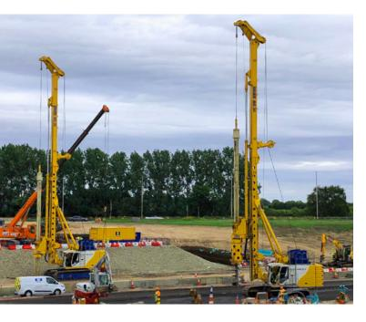
Specifically, Bauer was required to install 124 no. abutment CFA piles (62 per abutment), each measuring 900 mm x 13 m, and 60 no. pier rotary bored piles, each measuring 900 mm x 16 m. 2 no. preliminary test piles and 2 no. working test piles were also required.
