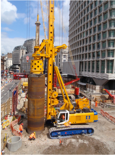
BAUER Technologies on site at Tottenham Court Road
