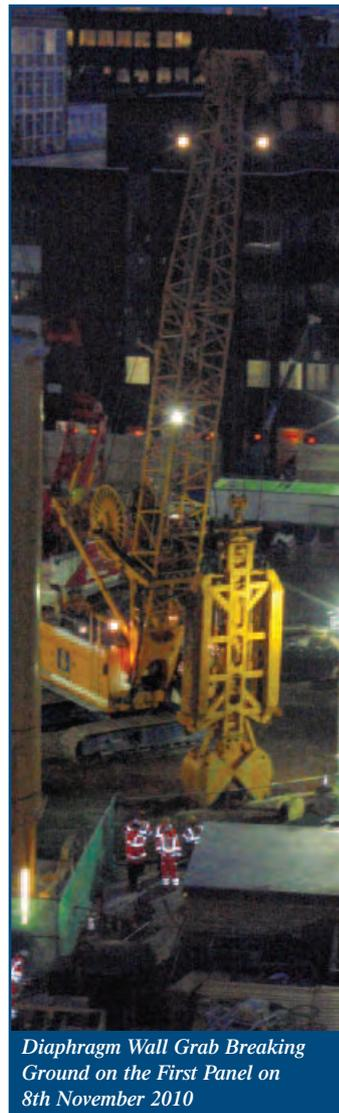
Diaphragm Wall Grab Breaking Ground on the First Panel on 8th November 2010
