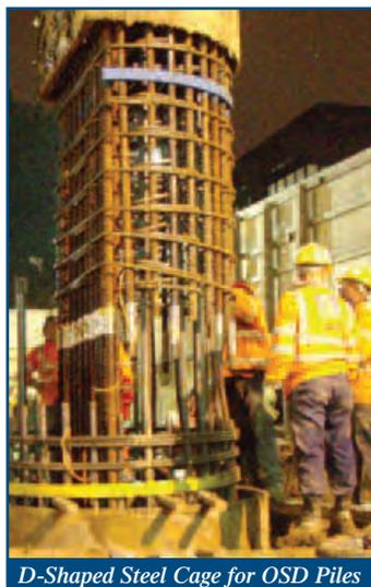
D-Shaped Steel Cage for OSD Piles
