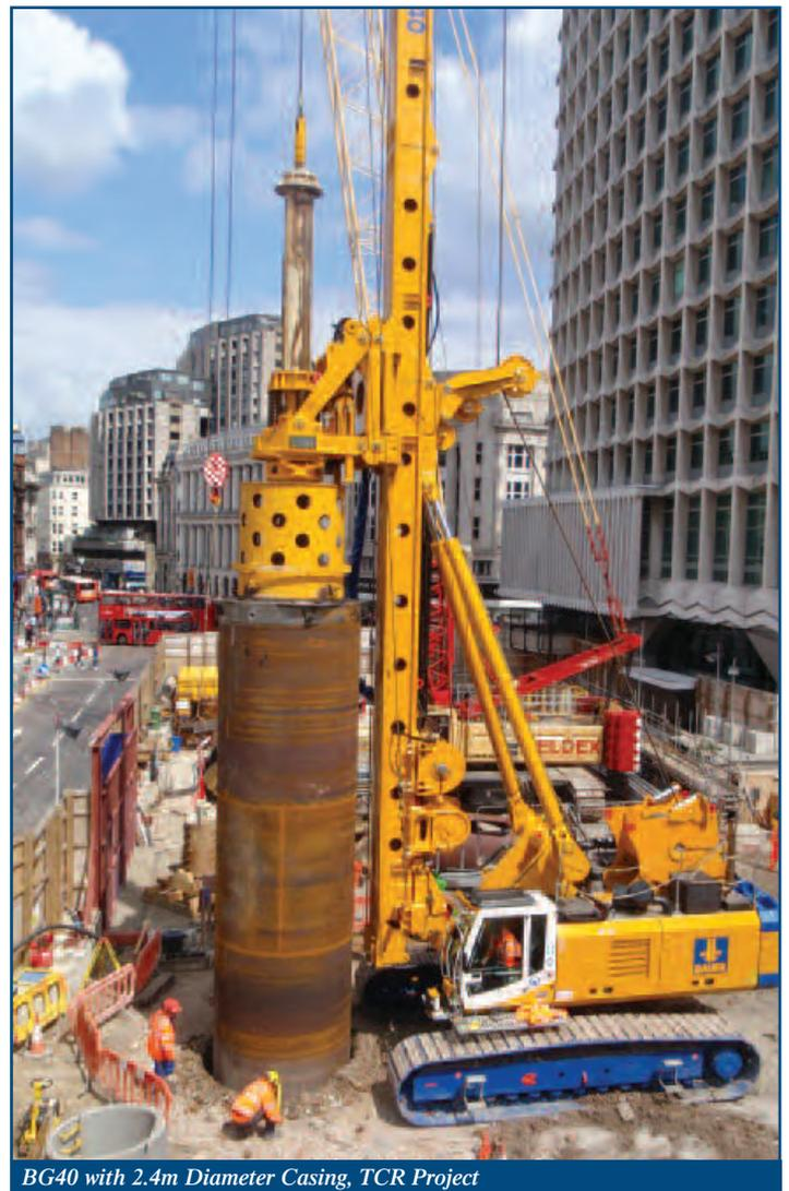
BG40 with 2.4m Diameter Casing, TCR Project
