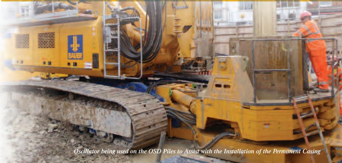
Oscillator being used on the OSD Piles to Assist with the Installation of the Permanent Casing
