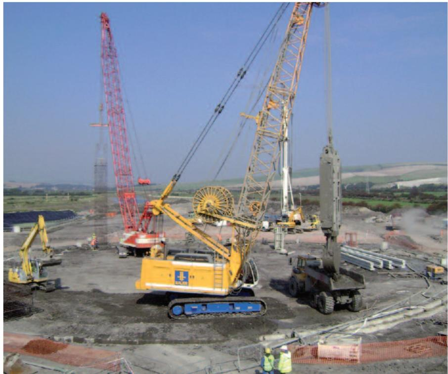
*Excavation with BAUER grab and reinforcement installation with service crane*
