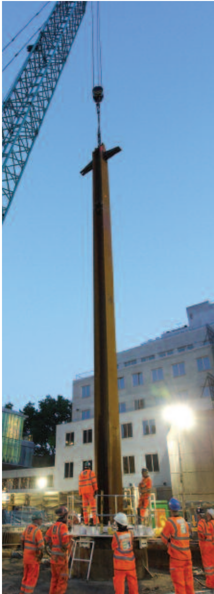
Plunge column works
