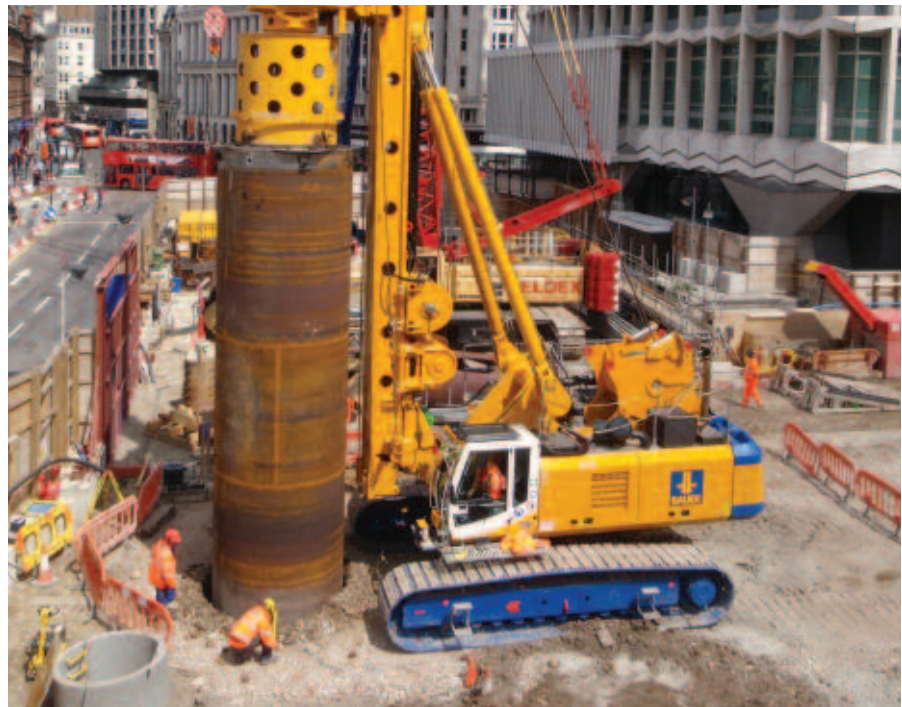
BG40 Piling Rig
