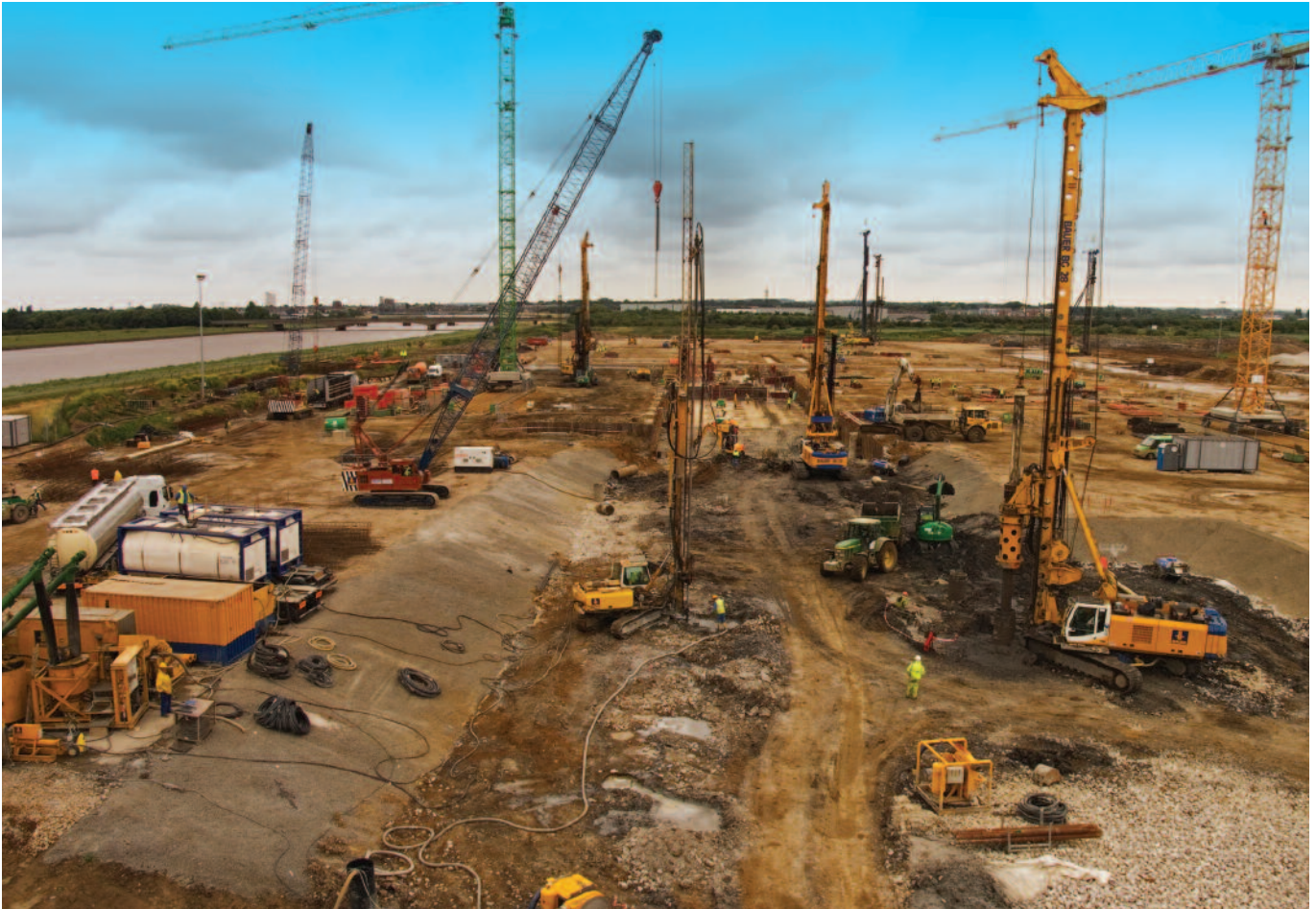
BAUER on site with 3 BG Drilling Rigs and 1 Jet Grouting Rig
