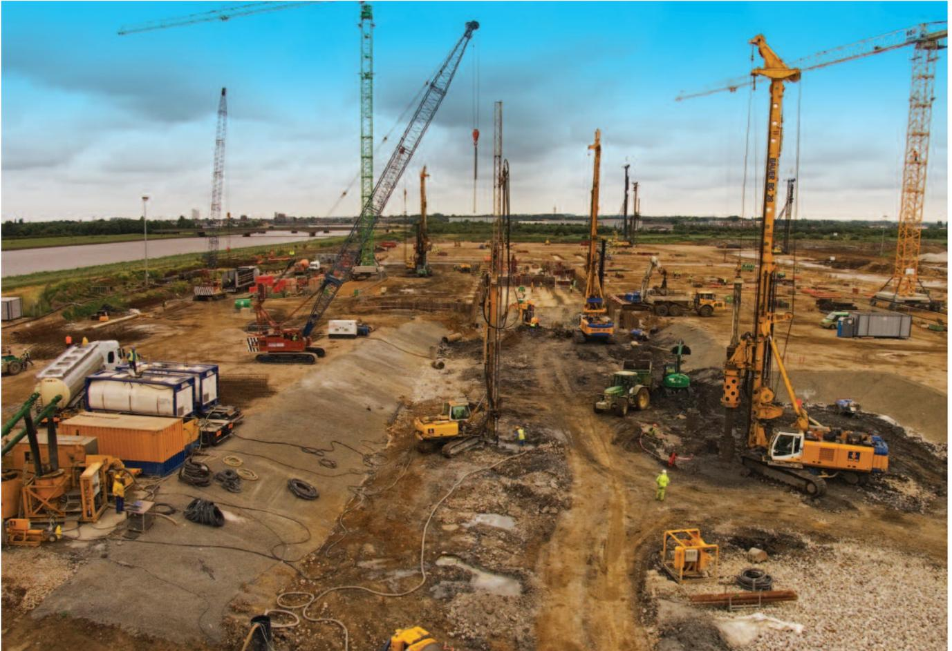
BAUER on site with 3 BG Drilling Rigs and 1 Jet Grouting Rig
